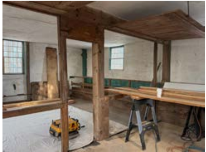
Original floorboards in place while work continued on upgrading boards replaced over the years.
