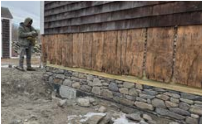
The raised foundation of the building was faced with fieldstone.
