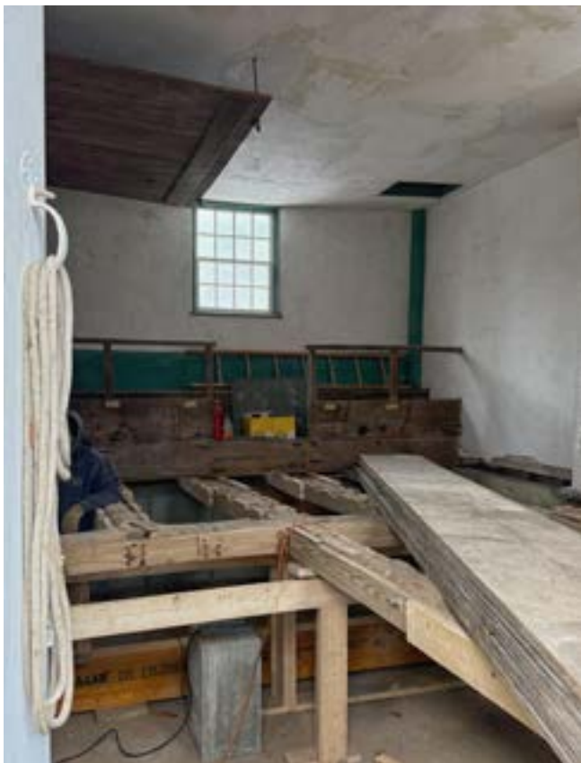
Meetinghouse interior with the floorboards removed and the new supports in place.
