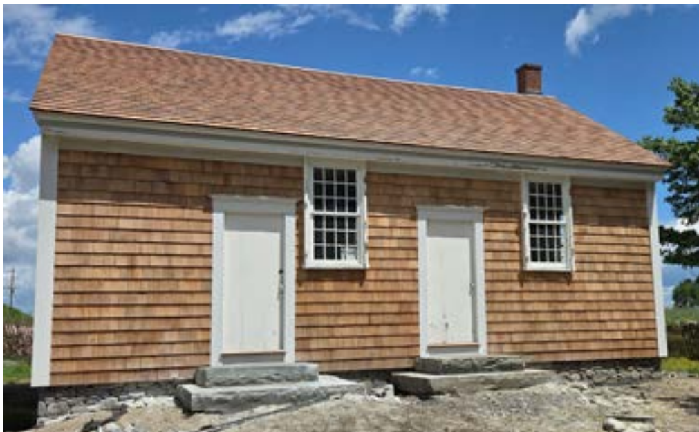
Sides and roof reshingled and the granite steps installed.
