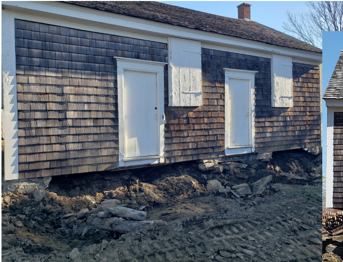
Dig out the old foundation.
