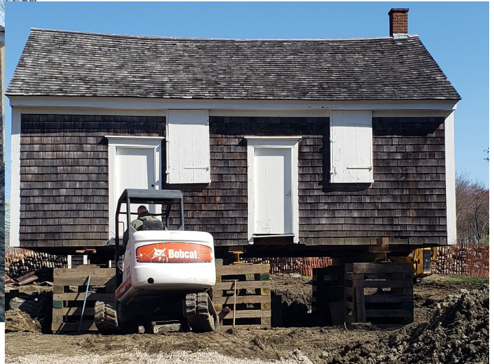
Lift and brace the building..
