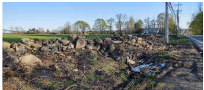
The dismantled wall in April.
