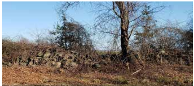
The wall in February before clearing began.
