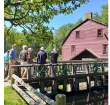
The sluiceway at the Gilbert Stuart House.
