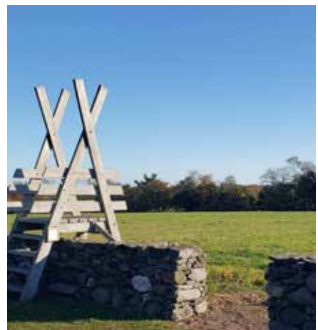
(right) New opening in wall next to stile
