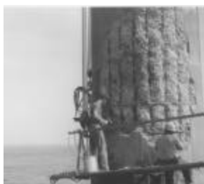
Jamestown Bridge maintenance
